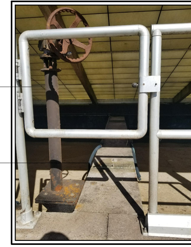
PHOTO 2 SCUM TUBE HANDWHEEL ACTUATOR
