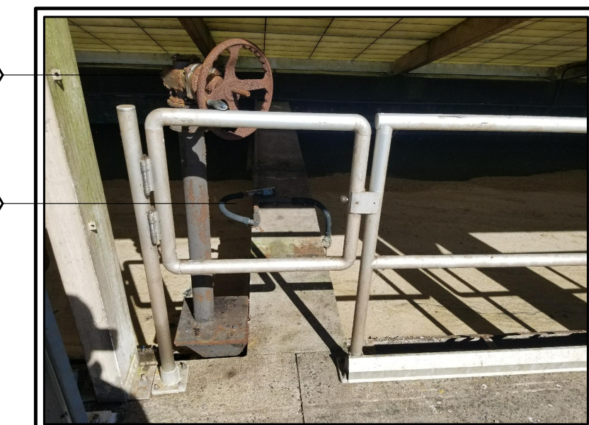
PHOTO 5 SCUM TUBE HANDWHEEL (TYP)
