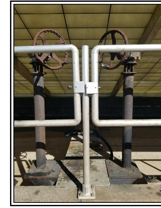
PHOTO 1 SCUM TUBE HANDWHEEL ACTUATORS
